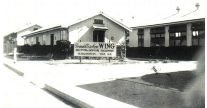
Demobilisation Building at Sandgate
